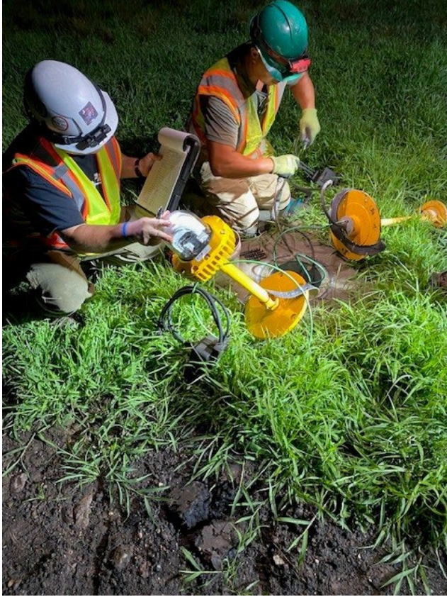
Installation of new LED runway elevated light fixture (left)
