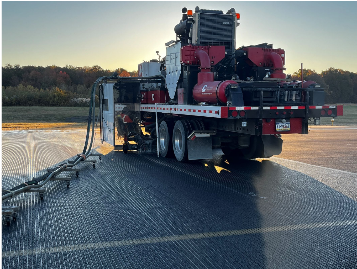
Grooving Operations on the Runway Proper
