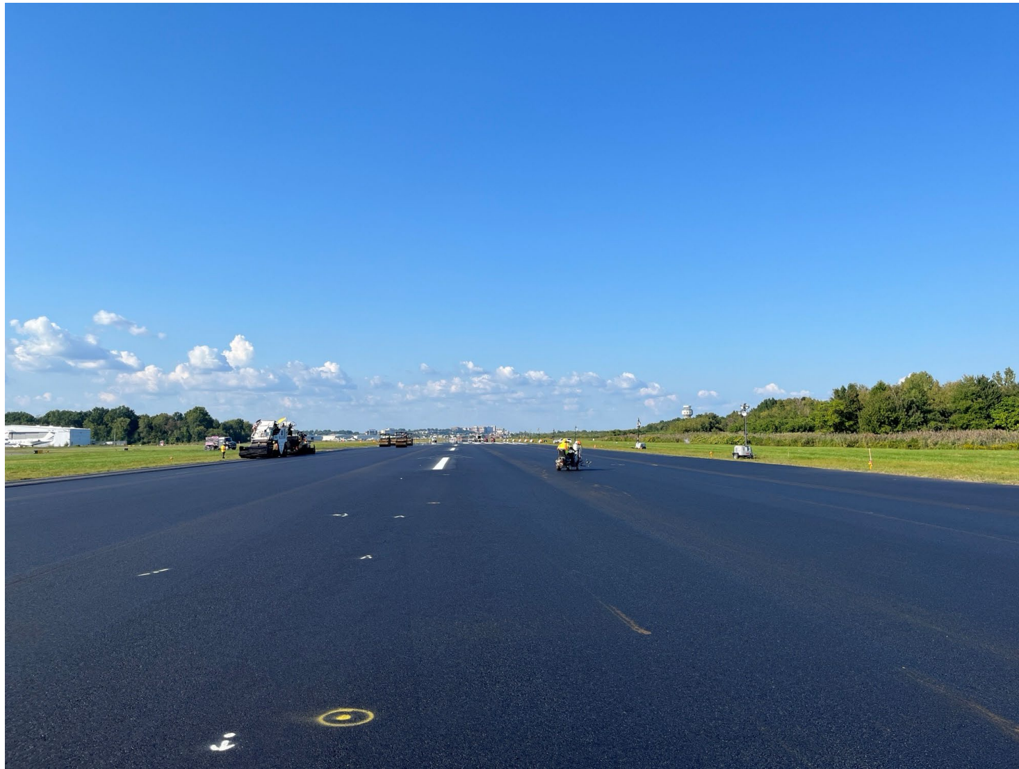
Runway Proper Asphalt Top Course
