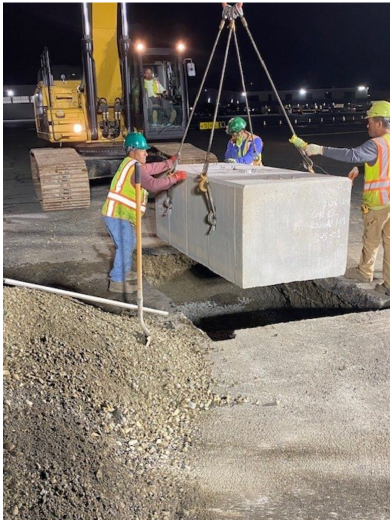
Sign Foundation and Cabinet Installation
