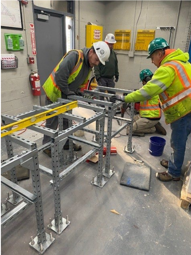
Preparation of elevated regulator platforms (left)
